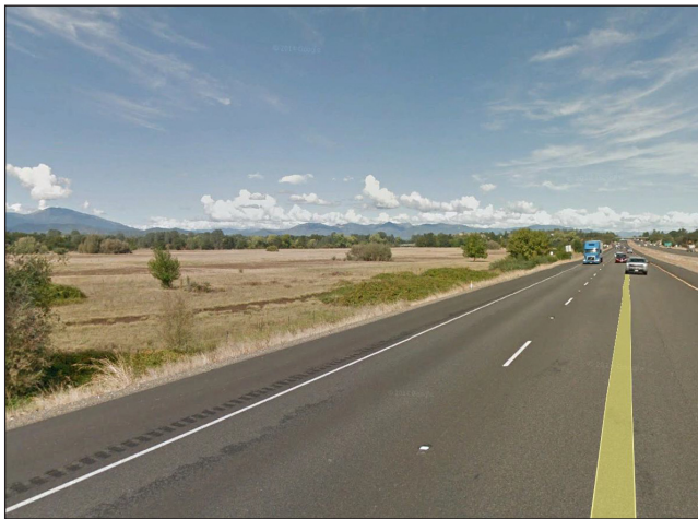
VIEW B - Facing northwest toward the Strawberry Fields Site.
