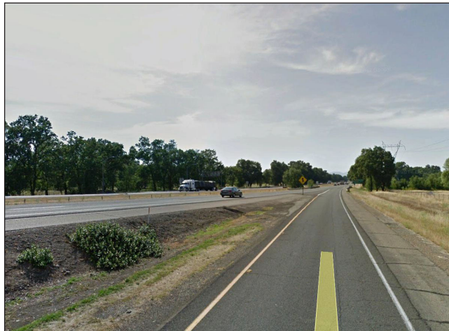
VIEW B - Facing northwest toward the Anderson Site.
